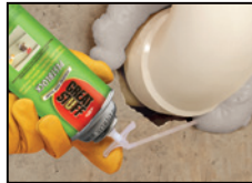
PVC pipe penetration
