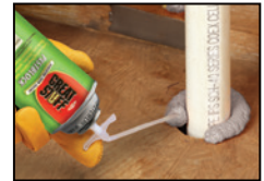
PVC pipe penetration
