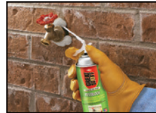
Water faucet penetration
