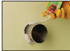
Dryer vent penetration
