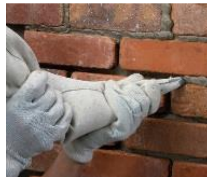
Installing Thin Brick and filling in joints
