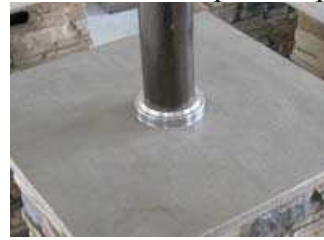
Figure 2-1 Assemble the cap to the post.
