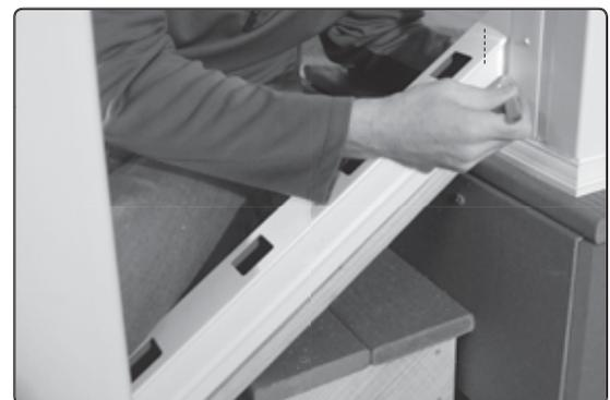
**4** Measure angle – take rail to chop saw and measure angle. Set saw and record angle. (NOTE: Do not cut here. This is for acquiring measurements.)
