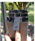
Remove: Post Caps\* and Channel Covers\* from 2 posts. <u>Determine</u>: Line, End, or Corner\* posts. <u>Measure</u>: 46" down from post top. <u>Insert</u>: Bracket\* through post, down inner Channel Slot\* to 46" mark Secure: Bracket short side down, with self tapping screw\*.
