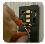
The wiring must be connected U to a transformer with a voltage of 8VAC - 24VAC and an internal doorbell or resistor.
