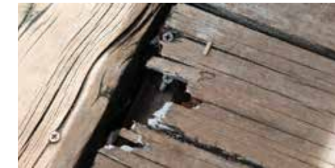
Shown Above: Ipe (Brazilian Walnut) Hardwood decking installed with face driven screws.
