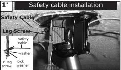
For Canadian installation and for USA fan and light kit combinations over 35 lbs, in both flush and downrod modes the safety cable must be installed into the house structure beams using 3" lag screws, washers and lock washers provided. Make sure that when the safety cable is fully extended the lead wires are longer than the cable and no stress is placed on the lead wires. **Note**:If Installing The Secondary Support Safety Cable in the U.S., Do Not Remove Knockouts In The Outlet Box.
