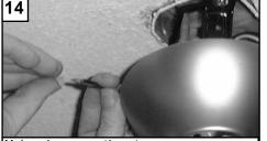
Make wire connections to power source using wire nuts provided. Make sure that no filiments are outside of the wirenut. After making the wire connections, the wires should be spread apart with the grounded conductor and the equipmentgrounding conductor on one side of the out let box and ungrounded conductor on the other side of the outlet box.
