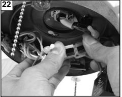
Connect plug from fan to switch housing plug. Match the color strips on the plugs.
