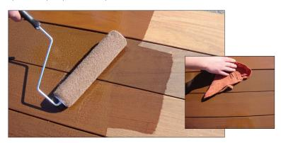
**Brush, Roller & Rag Application:** For the best results, utilize a high quality 3/8" nap roller, pad applicator or stain brush. To minimize lapping, maintain a wet edge lengthwise and do not break in the middle of boards. One coat is sufficient for most applications. Always apply oil onto the boards parallel to the grain of the wood. **NOTE: Product not absorbed into the wood within 30-45 minutes must be thoroughly removed.**
