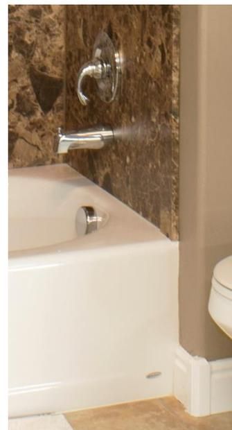
Vertical trim installed to top of tub
