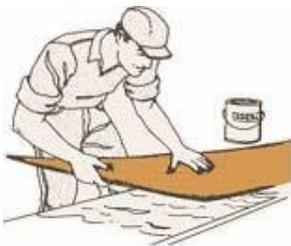
Adhesive application may be used to apply Hardboard requiring both adhesive and nails.
