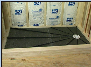
Pre-Pitch™ Standard and Extended installed in rough-in.
