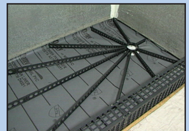
Quick-Pitch® Standard and Extended and Kirb-Perfect® installed.
