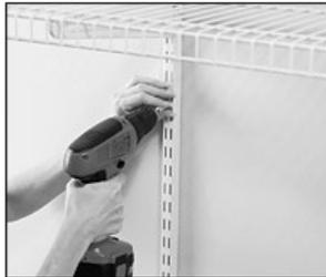
Each Standard must be secured to the wall with one screw at the closest hole to the center of the Standard. When using toggle bolts, remove toggle, put bolt through Standard and re-attach toggle to bolt before placing Standard on track.
