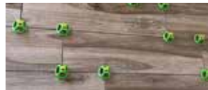
Large format Tile floor Install
