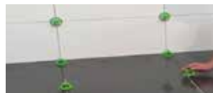
Floor & Wall Tile Install
