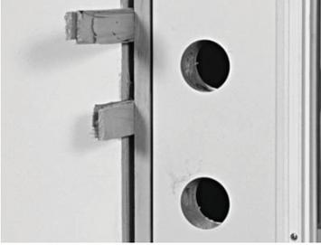
Shim behind the latch-side jamb approximately 8" from the top and bottom of the frame. Install shims until there is an even 1/8" gap between the jamb and the edge of the door slab along the whole length of the door. Shim behind the latch-side jamb just above and below the dead bolt hole, maintaining the 1/8" gap. Pull the weather-stripping away from the jamb and screw 3" installation screws through the jamb and shims and into the stud.
