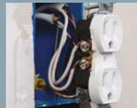
Screw terminal where a wire is connected to a receptacle may become loose as it is pushed back into the work box
