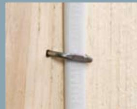
Hammering electrical cable staples too tightly into studs during rough wiring
