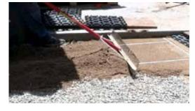
IMPORTANT: Do not use sand to level depressions in the base layer. Instead, add base material to level the area.
