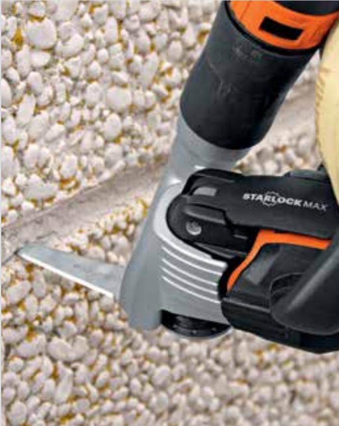
Dust extraction is used when working with hazardous grout materials (e.g. PCB).
