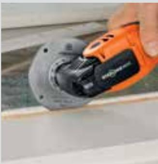
Cutting through nails on window bars.
