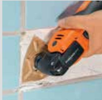
Sanding tile adhesive flush before filling in again.
