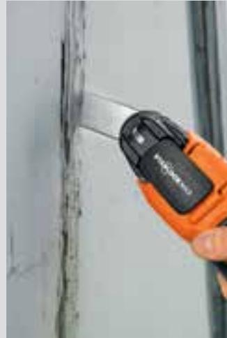
Removing flexible grout sealants in building construction and civil engineering.
