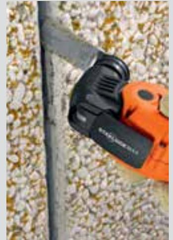
Roughening the mortar flanks before filling in again.
