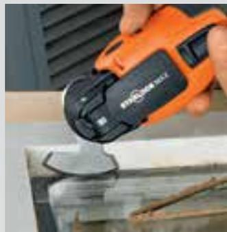
Cutting out putty-mounted insulation glass windows.
