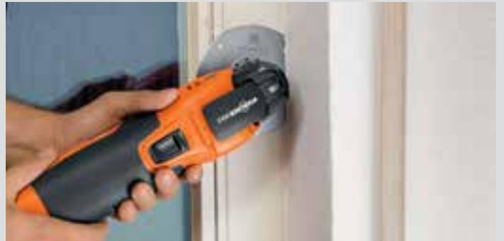
Cutting through metal bracings when dismantling old windows.
