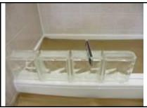
**2.3** Place an "L" spacer and a "T" spacer on the bottom of the first glass block. Place the glass block on the shower base curb. Sit a level on top of the glass block and trim the tabs of each spacer until the glass block sits level on the curb. Repeat this procedure for the first course of glass blocks. Use the modified "L" spacer at the wall, three modified "T" spacers between the glass blocks and flat spacer under the EndBlock® Finish Unit.
