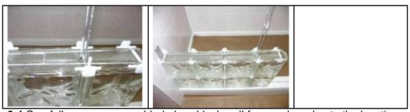
**3.4** Carefully remove assembled glass block wall from curb and note the location of each modified spacer under the first course of glass blocks.
