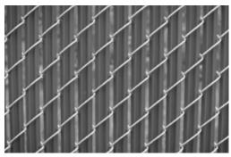
2. Continue inserting Channel-lock privacy slats individually until desired section is covered
