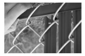
1. Insert Channel-lock privacy slat tapered end up into fence channel, until bottom of slat reaches the ground.
