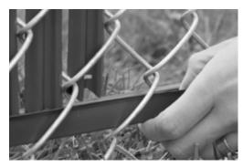
3. Insert Channel-lock privacy slat through top of fence with tapered end being down. Gently slide Channel-lock slat downwards until locking slit securely locks into locking channel.
