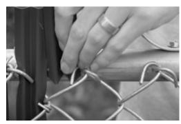
2. Then insert locking channels into bottom of fence, one space above bottom of fence line.
