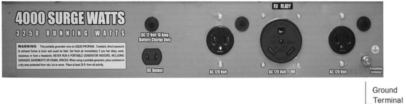
Figure 3 - Attaching the Grounding Wire to this Generator
