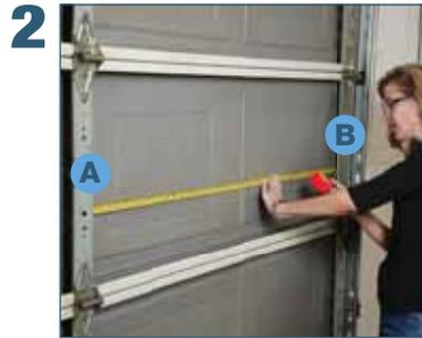
Measure length between vertical rail A to the inside edge of vertical rail B.
