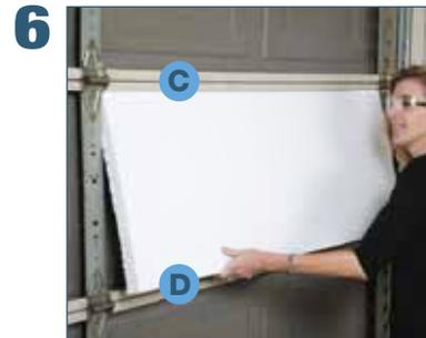
Insert the insulation sheet between horizontal rails C and D with the channeled or grooved side facing the garage door.
