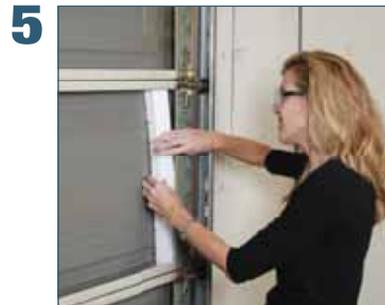
Insert the excess insulation behind the vertical rails.
