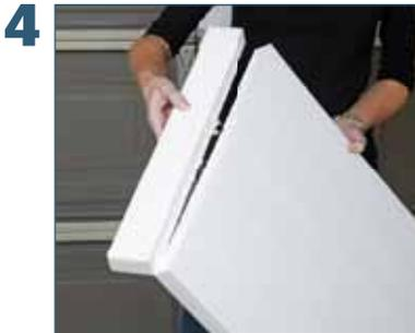
Break off the insulation where cut.
