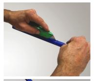
1. Cut and fold back plastic cover to reveal the copper tube
