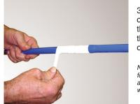
3. When the joint is complete and cool, replace the plastic coat and wrap the joint to give continuity of protection
