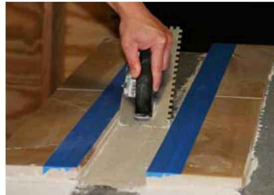
Apply a thin layer (bond-coat) of one of the recommended thin-sets (page 6).
