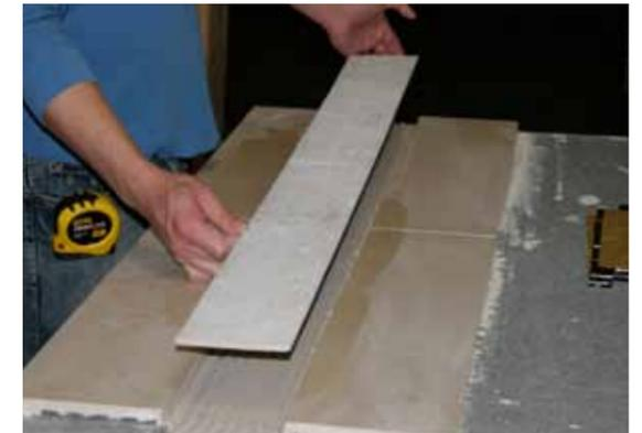
Use one of the recommended thin-sets (page 6) to install a piece of  $\frac{1}{4}$ " or  $\frac{1}{2}$ " cement board. Use a notch trowel size and cement board thickness that will render the desired substrate depth. Cure a minimum of 24 hours.
