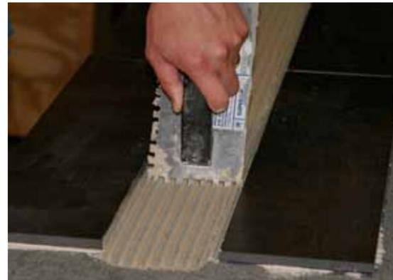
Use one of the recommended thin-sets (page 6) and a notch trowel to apply a layer of thin-set. Use a notch trowel size that renders the desired substrate depth once the notches have been flattened.
