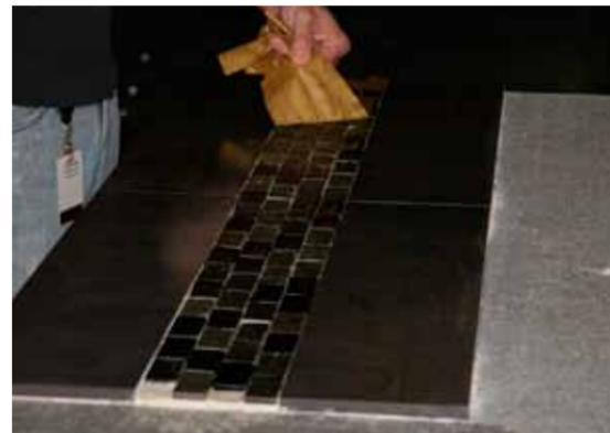
After the flattened layer of thin-set has cured for a minimum of 48 hours, install and grout the tile per the instructions on pages 15-18.
