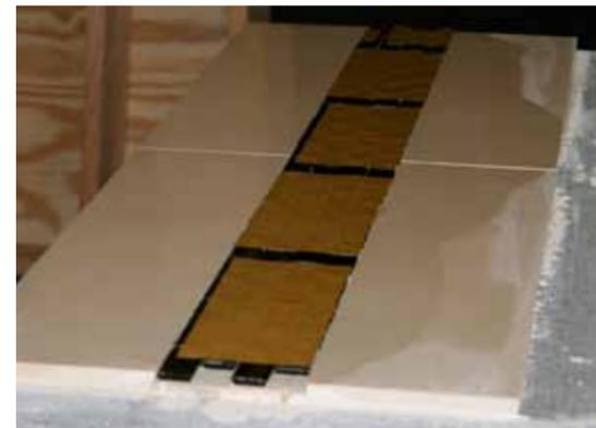
After the installed cement board layer has cured for a minimum of 24 hours, install and grout the tile per the instructions on pages 15-18.
