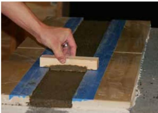
While the bond-coat is still tacky, apply a cement mortar bed (sand & cement mixture per ANSI A108.1B). Screed the cement mortar bed to the desired substrate depth and cure a minimum of 7 days.
