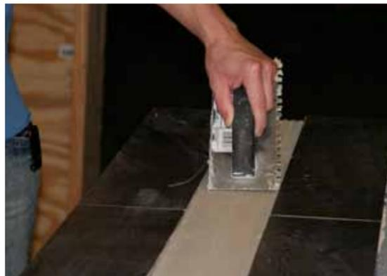
Without removing any thin-set, flatten the thin-set notches. This step should yield a smooth consistent setting bed of uniform depth. Cure for a minimum of 48 hours.
