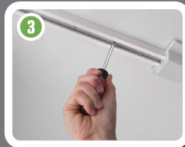
Attach track to ceiling.
