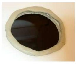
Figure 5. Installed drain assembly showing excess plumbers putty: If using caulk, tighten the nut only part way until caulk starts to compress and starts to squeeze out. Allow the caulk to skim over then tighten the nut completely.
