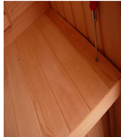
FIG 10 Securing Benches with screws
