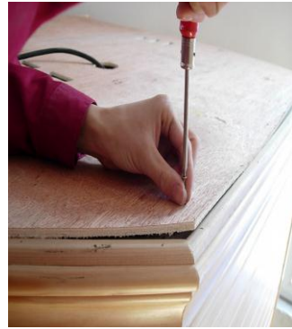
FIG 18.1 Screw down Roof Cover
