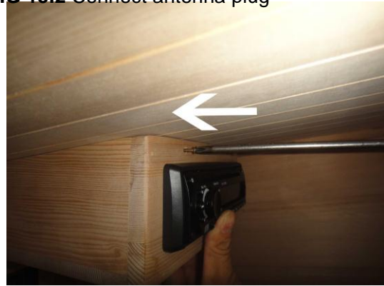
FIG 15.4 Screw wood housing to sauna room
