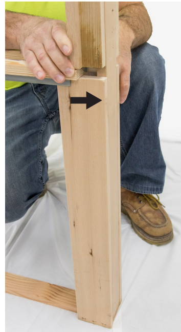
Flush aligned for rough opening
