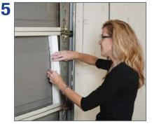
Insert the excess insulation behind the vertical rails.
