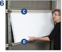
Insert the insulation panel between horizontal rails C and D with the channeled or grooved side facing the garage door.
