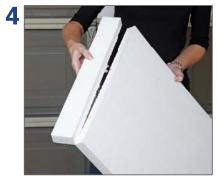
Break off the insulation where cut.
