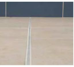
RONDEC edging profile and corner piece accessories used to used to finish the tile edges on the wall. DILEX-EKE PVC movement joint profile separates individual tile fields at floor-to-wall transitions and inside wall corners. DILEX-BWB PVC movement joint profile installed in the floor.
