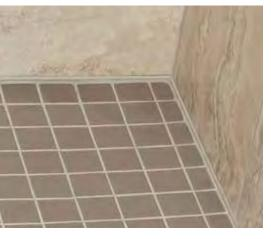
RONDEC bullnose profile used to finish the tile edges on the wall and tile base. DILEX-EKE PVC corner movement joint profile in classic grey used to create a seamless transition between the shower walls and floor.
