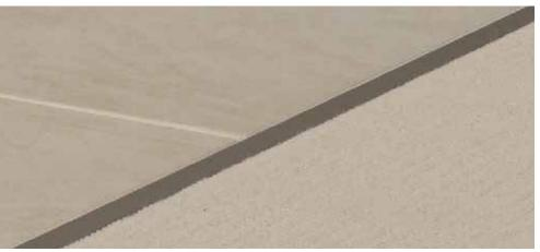
RENO-TK floor profile used to create a smooth transition between the tile and carpet.
