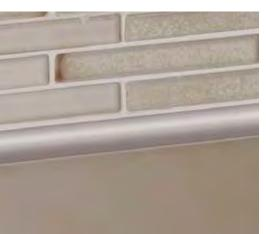
RONDEC-STEP edging profile applied to the sink rail. RONDEC bullnose profile and large radius sink corners used to produce the tiled-under sink. DILEX-AHK cove-shaped profile used to create a smooth transition between the countertop and backsplash.
