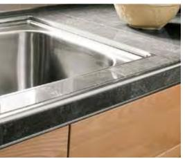
RONDEC bullnose profile and corners used to finish the countertop trim and tile edges of the backsplash. RONDEC was also used to produce the tiled-under sink. RONDEC-CT double-rail edging profile applied to the sink rail. DILEX-AHK cove-shaped profile used to create a smooth transition between the countertop and backsplash.
