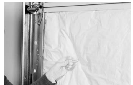
Install Retention Clips
