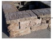
**Step 4**: Install the caps (8 units). Start at a corner and place a cap on the fire pit leaving approximately a 1" overhang. Continue placing caps around the fire pit making slight adjustments as needed to get the caps in place. The inside diameter of the caps needs to be a minimum of 28". Remove the caps one at a time and adhere each cap to the blocks below with a quality concrete adhesive.
