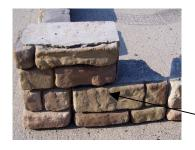
**Step 3**: Install second course of blocks (10 units). Place a corner block on top of the bottom corner block staggering the intersection of two blocks on the course below. Continue around the fire pit making slight adjustments as needed so that the edge of the blocks fit tightly. Remove the blocks one at a time and adhere each block to the blocks below with a quality concrete adhesive.
