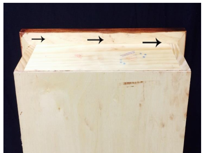
Image 4 Apply Construction Adhesive
