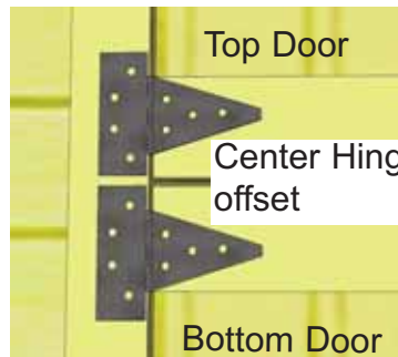
Top and Bottom Hinges centered on door trim.
