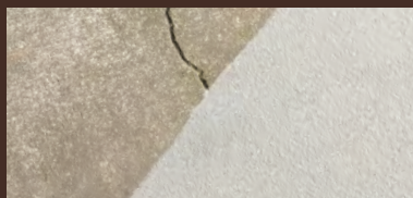
REFINISHES CONCRETE RESTAURA SUPERFICIES DE CONCRETO
