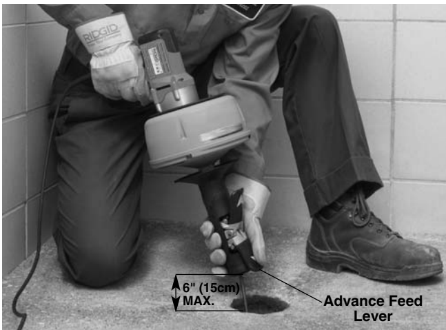
Figure 10 – Feeding Cable With AUTOFEED
