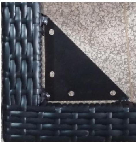
Top side of frame
