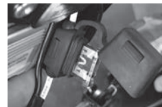
THE 30 AMP MAIN FUSE IS LOCATED BEHIND THE FUSE PLATE COVER IN A WEATHER PROOF RUBBER FUSE HOLDER
