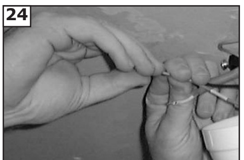
24 Make wire connections to power source using wire nuts provided. Make sure that no filiments are outside of the wirenut. After making the wire connections, the wires should be spread apart with the grounded conductor and the equipment-grounding conductor on one side of the outlet box and ungrounded conductor on the other side of the outlet box.
