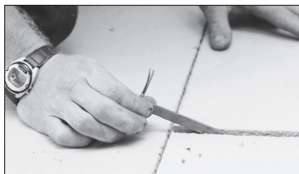
Maintain 3/16" Spacing Between Panels Read All Instructions Carefully
