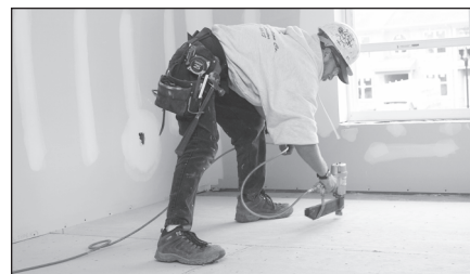
Nail and Finish Floors and Walls
