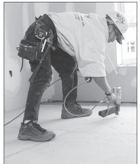
Nail and Finish Floors and Walls
