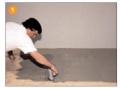
Using a thin-set mortar that is suitable for the substrate, apply the thin-set mortar (mixed to a fairly fluid consistency, but still able to hold a notch) using a 1/4" x 3/16" (6 mm x 5 mm) or 5/16" x 5/16" (8 mm x 8 mm) V-notched trowel.
