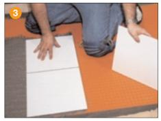
Tile can be installed over Schluter®-DITRA immediately; no need to wait for the mortar to cure. Using a trowel that is appropriate for the size of the tile, apply the bonding mortar (unmodified thin-set mortar) and solidly embed the tiles in the setting material, making sure to achieve full coverage.
