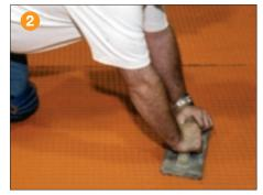
Apply Schluter®-DITRA to the floor, fleece side down. Work DITRA into the mortar, using a float or screed trowel in such a way that the fleece of the DITRA is solidly embedded in the bonding mortar throughout its entire surface (please observe the open time of the bonding mortar). After applying DITRA, lift up one corner to check the fleece for full mortar coverage. For joining sections of DITRA, simply abut end and side sections of adjacent sheets.
