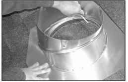
3. Locate base opening between rafters and mark hole(s) to be cut. Locate rafters by tapping roof.
