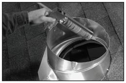
8.Seal the adjusting seam and the base/elbow connection seam on inside with roofing cement. Seal locking clamp holes and all exposed nails with roofing cement.
