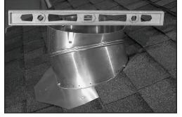
6.Rotate top of elbow to level position by turning counter clockwise.
