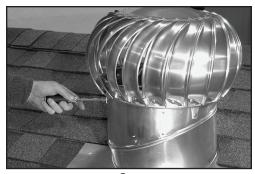
9.Position Whirlybird<sup>®</sup> on the base. Line up the predrilled holes in the brackets and elbow and fasten with sheet metal screws.
