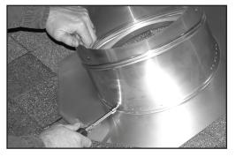
2.After turning bottom of elbow clockwise to align roof pitch number with indicator line on flashing. Place 3 screws through holes that line up with predrilled holes in base.
