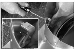
7.Place locking clamp across seam and tighten as shown, with included screw.
