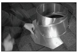
5.Slide top half of flashing under shingles. Secure with nails at top, sides and bottom.
