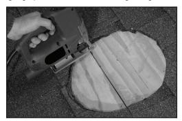
4.Cut hole as marked. Seal around entire perimeter of hole with roofing cement.
