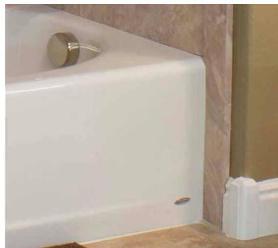
Vertical trim installed outside tub, and contour cut to match tub shape
