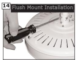
Remove the 2 yoke set screws as shown above.
