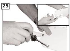
Place blade holders onto blades aligning holes in blade holder with holes in blade. Make sure that the side of the blade you select is facing downward. Install 3 screws and fiber washers to back side of blade as shown. Tighten screws securely. Repeat this process 4 more times until all blades are assembled.
