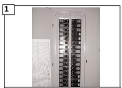
Before you begin installing the fan, Switch power off at Service panel and lock service disconnecting means to prevent power from being switched on accidentally. When the service disconnecting means cannot be locked, securely fasten a prominent warning device, such as a tag, to the service panel.
