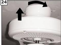
Lift fan to mounting bracket, aligning the "L" shape holes with the scresws on the mounting bracket. Turn the fan clockwise to lock in position. Install the 2 canopy mounting bracket screws from the hardware pack and tighten securely.
