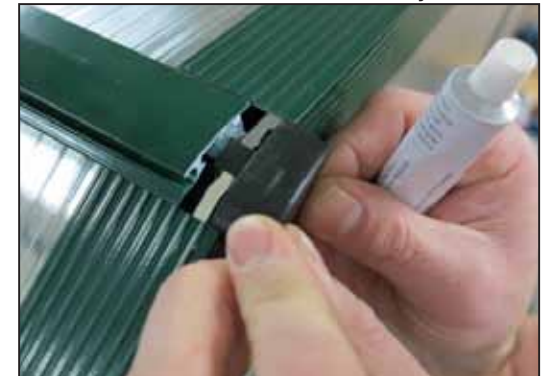
The two profiles should be flush at ends when installed correctly.
