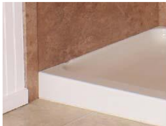
Vertical trims installed outside shower base
