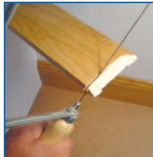
**Step 1** - Cut the first piece of trim to length and position it on the wall. Use straight cuts, no angles.
