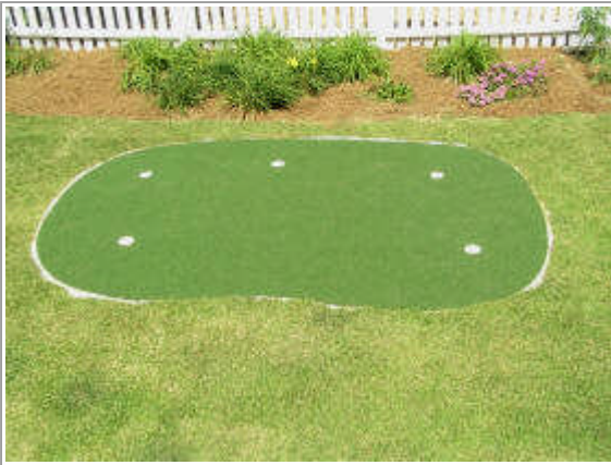
(16) Roll out green and inspect contours and level cups. Cups can be leveled by stepping gently on their edges.
