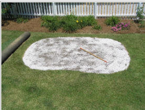
8) Create a gentle crown in the center for drainage with a leveling rake or 2x4 and rake the area smooth. No indentations should be present.
