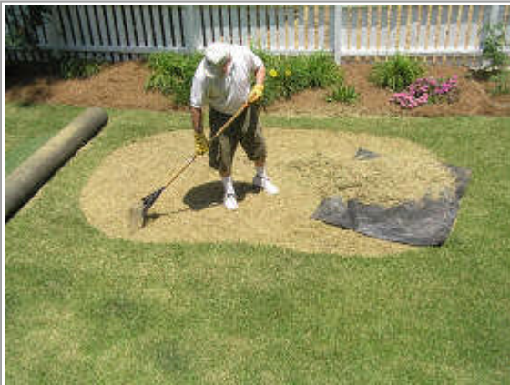
6) Rake or blow cuttings from outlined area, and cut ridges or roots if necessary. Fill any indentations
