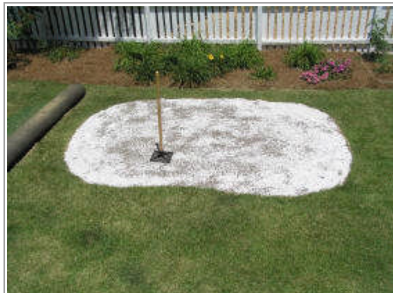
9) Compact the base with a hand tamper. A base of #8 crusher rock mixed with paver sand is used because it is resilient and holds it's shape better than pure sand.
