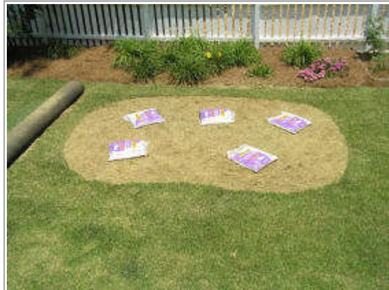
7) Add up to 2 lbs. of base for every square foot of green. #8 crusher rock mixed evenly with sand (1 to 1) is recommended for base
