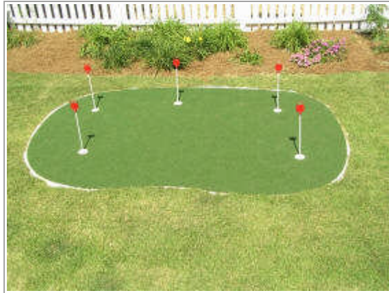
(17) Clean and add markers or flags (optional). Surface can be raked (leaf or carpet rake), blown, vacuumed with a beater bar or hosed off or gently pressure washed.
