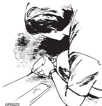
Once you've found the location in the partition wall, you must center the access hole in the middle of the wall. Measure half the thickness of the wall and mark the center of the wall where you will drill the access hole. If you cannot see the plate, you can determine this measurement from upstairs. At the nearest doorway, measure the thickness of the wall, including the baseboard.
