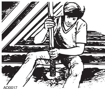
For a basement installation, assemble the tubing to the inlet flexible tubing in the same way and insert it into the access hole. A basement inlet line is necessarily shorter because it must only reach 18" from the floor to the inlet. Most of the time, basement inlet lines are more easily installed by two people after the inlet hole has been cut in the interior wall. See "Wall Inlet Installation."
