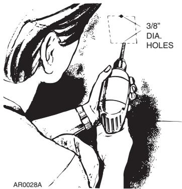
Also drill four pilot holes in the four corners of the marked area. Make sure these holes are located inside the marked line. Then, using a utility knife, score along the inside of the marked line. For plaster walls, score the plaster deeply, being careful to stay inside the marked line.
