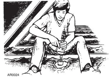
Now, use a flashlight to inspect the wall cavity through the access hole. Make sure no hidden obstacles will interfere with the tube installation. (If this inspection reveals an obstacle, find a new inlet location.) Repeat this procedure in your attic or basement until your access holes are drilled.
