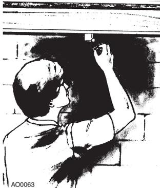
Attach the tubing to the joists or ceiling with either perforated metal or support strapping (support strapping is available from NuTone).
