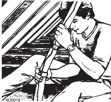
Whatever the case, insert the completed inlet line into the access hole and thread it down inside the wall. The inlet line should be long enough so that it extends above the joists in the attic; at this height, it can be easily connected to the branch and truck lines. When cutting the inlet tubing to length, remember that your inlet will be placed at 18" above the floor.
