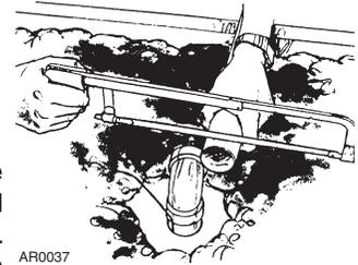
Bring the trunk line to the access hole you have drilled for the power unit's intake tube. Place a 90° elbow over the hole and cut the trunk line to fit into this final elbow. Allow 5/8" of tubing to fit into the elbow's collar. Connect the elbow to the trunk line so that it aligns over the intake access hole. You will make the intake tube connection itself after you have installed the power unit.
