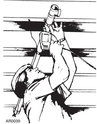
Make all branch line connections in the same way you would an attic installation. Make sure that all branch lines enter the trunk line at an angle that is at least levelled with the trunk line. Make sure all the fittings are oriented so the air flows toward the power unit. Complete the trunk line to the power unit location.
