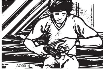
Tuck the 6" wire lead inside the flexible tubing so that it will not snag inside the wall.
