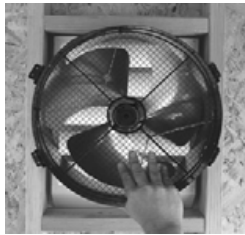
Fan be installed in the wooden frame
